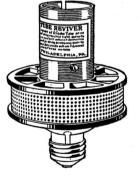
from the socket and should be entirely cured. The reactivator is made in two models, one for 199 type tubes and the other for the 201-A type.
