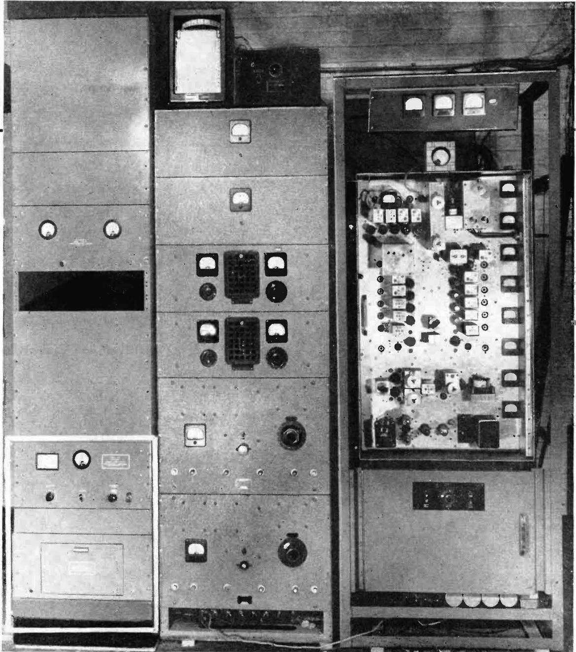
Size comparison between the Serrasoid modulator (outlined in white) and the original Dual-Channel modulator at the right. Center rack and upper section of left rack are used for other equipment. Photograph taken at the Armstrong f-m broadcast station W2XMN-W2XEA at Alpine, N. J. where the new modulator has been in service for six months
