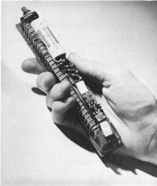
Fig. 41 - Close-up view of transistor phonograph oscillator.
