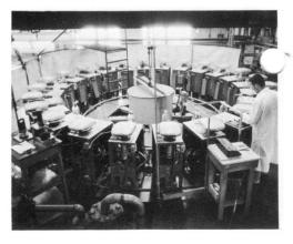
Each bulb is evacuated by means of mechanical and oil diffusion pumps in order to insure an even distribution of the vaporized aluminum. As the filament is heated in the vacuum, the aluminum slug melts, vaporizes, and then condenses on all surfaces inside the
